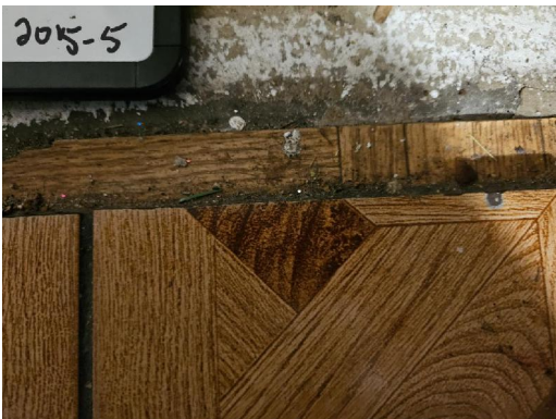
2015-5 Rolled Flooring/Mastic Interior Kitchen
