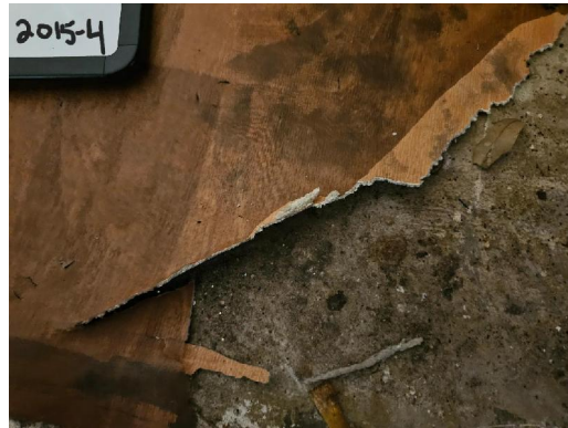
2015-4 Rolled Flooring/Mastic Interior Laundry Room
